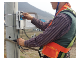
Work Belt on the telephone pole
